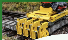
Rail and Sleeper Handling
