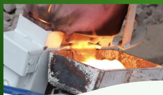
Aluminothermic Welding
